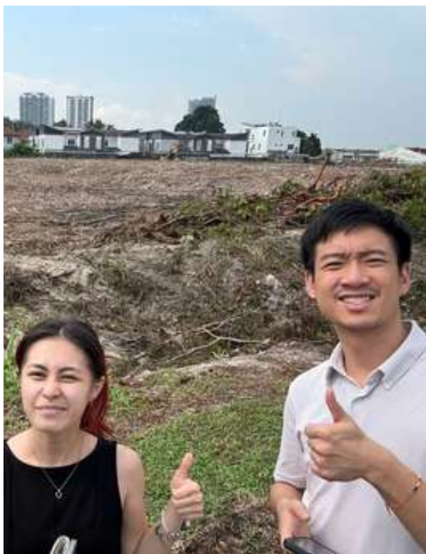
Land Clearing Works Steadily Underway as of June 2025
